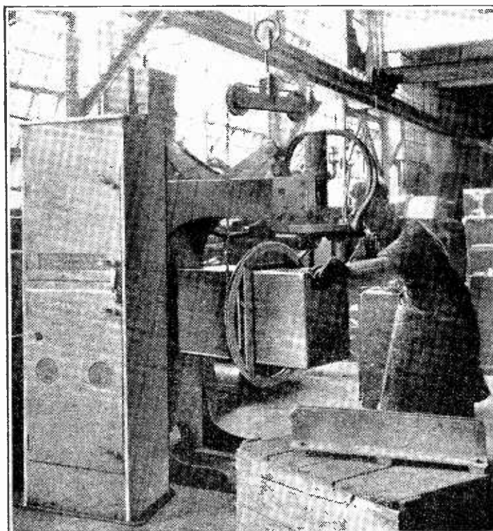
Photograph by courtesy of the Brush Thomson-Houston Company.
